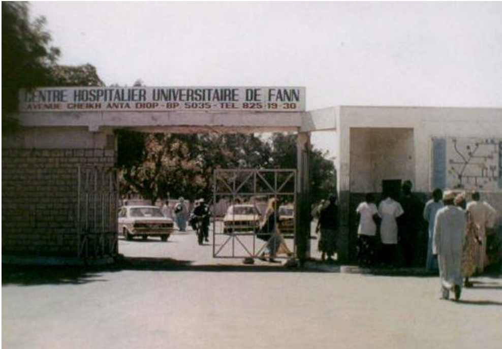
Figure 5 Image Showing the Front Entrance of Fann Hospital
