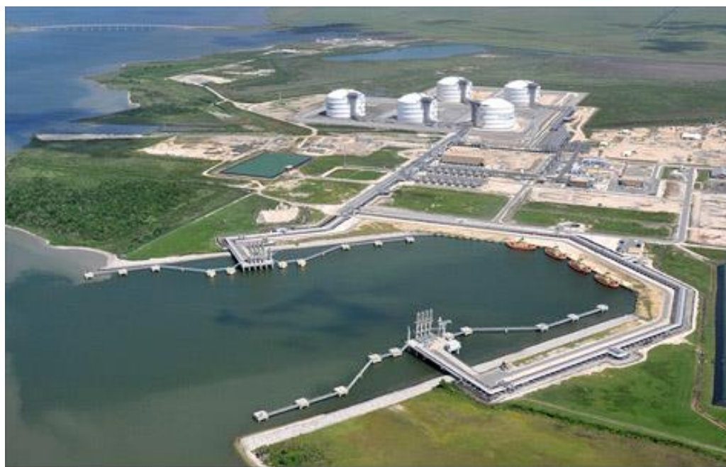
Figure 4: Photo of Sabine Pass
