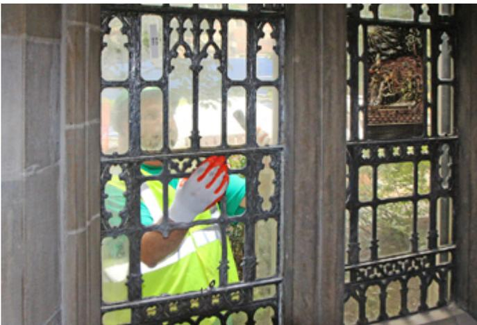
A worker in the Selin Courtyard removes a portion of the stained glass windows in the north aisle, so that the glass and lead elements can be restored. **Photo by Phil Handler, Fly on the Wall Productions**
