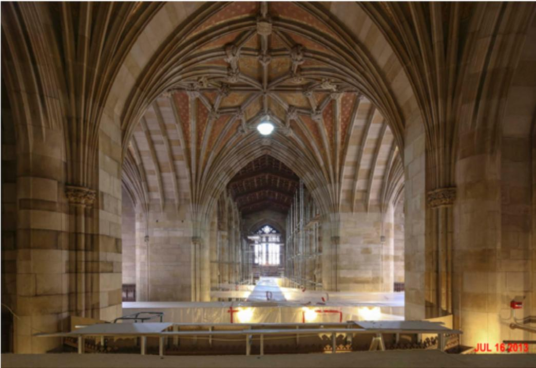
*Left:* A view of the nave interior looking from above the circulation desk towards the High Street entrance. Here, 50% of the scaffolding is installed; eventually scaffolding would fill the entire space up to the ceiling.
